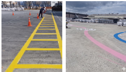
Safety Line Marking inside Storage Yards and Worksites
